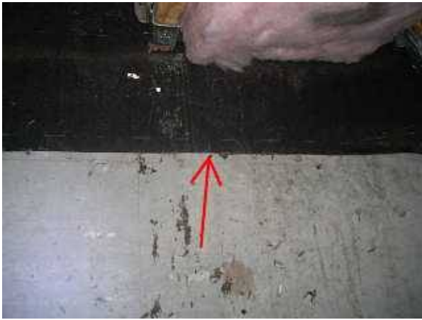
Photo 10 Tar paper covering vents at perimeter.
