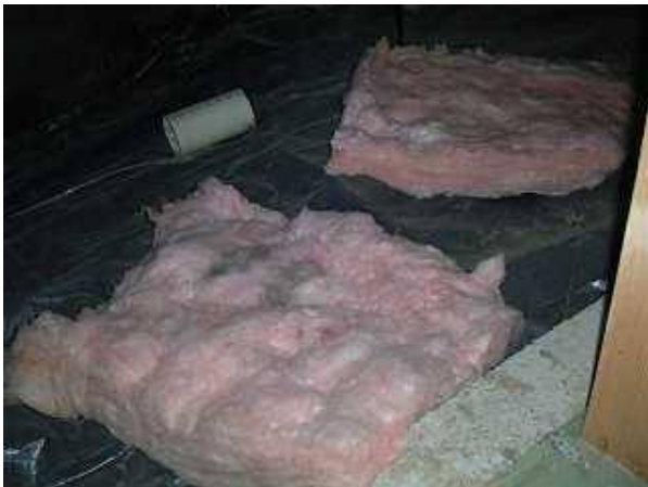
Photo 8 insulation on grade
