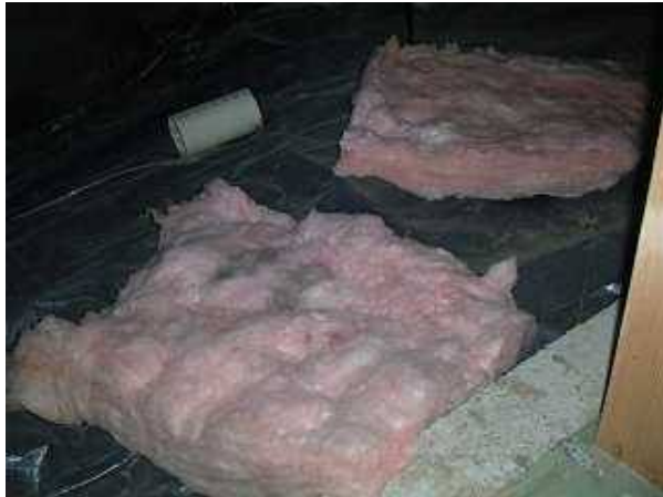
Photo 8 insulation on grade
