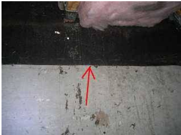
Photo 10 Tar paper covering vents at perimeter.
